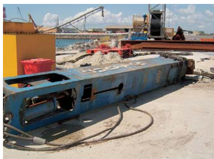
... and a hydraulic hammer
