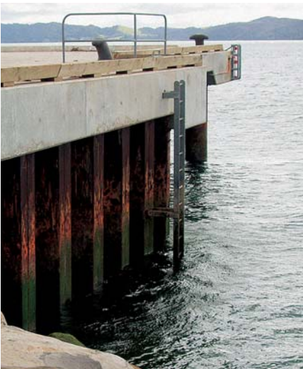
The 390-m wharf was completed with returning walls at each end
