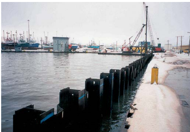
New sheet pile wall installed 1.5 m in front of the existing wall
