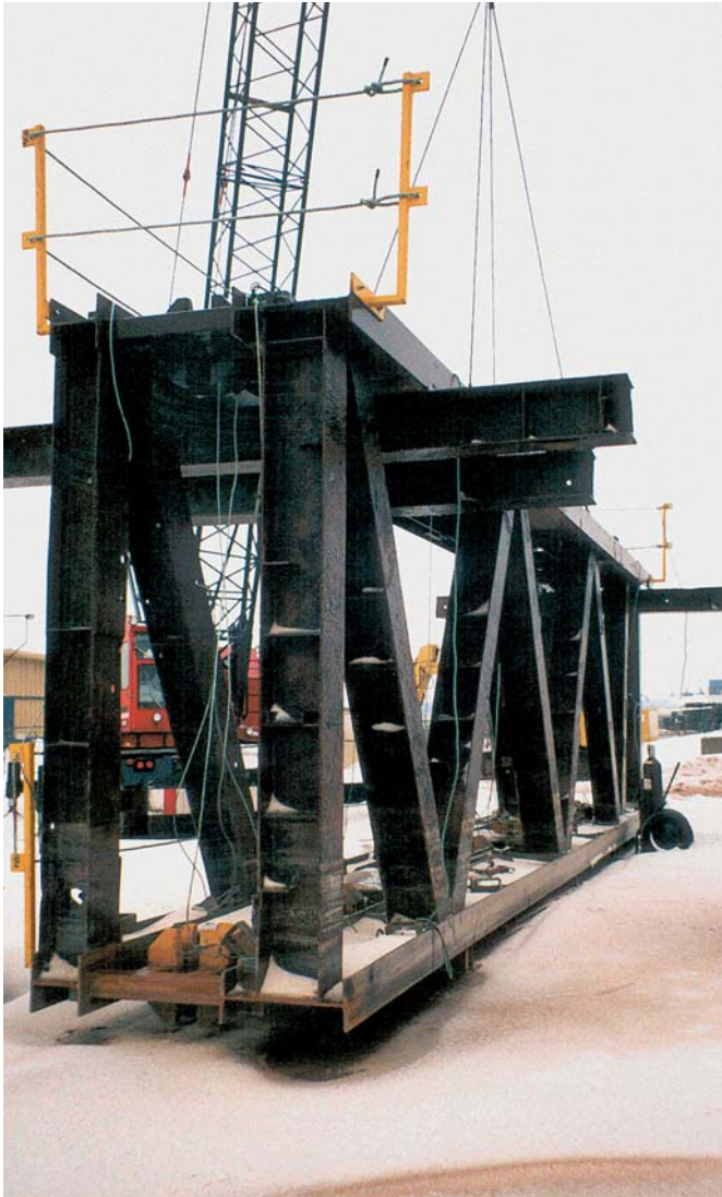
The two-level template ensures the king piles are correctly positioned for driving
